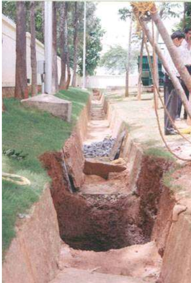
Recharge wells for storm water
