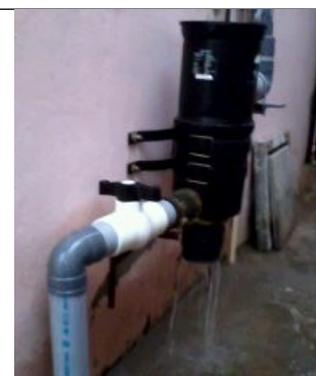
*Rejected water coming out from the bottom of the filter*
