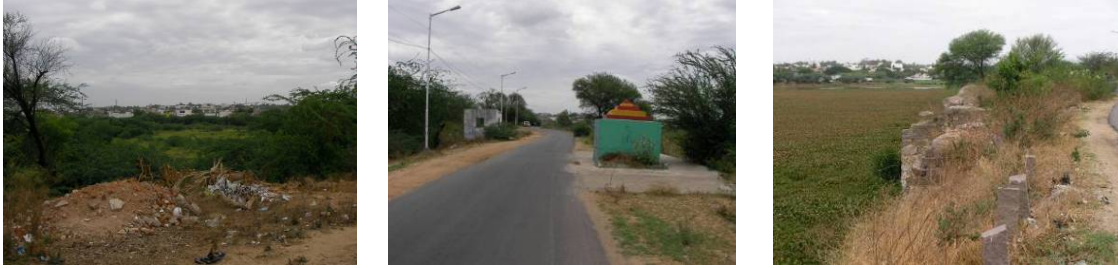
Figure 5: The divided lake: the dike of Maqbool nagar, the road, the old outlet sluice
