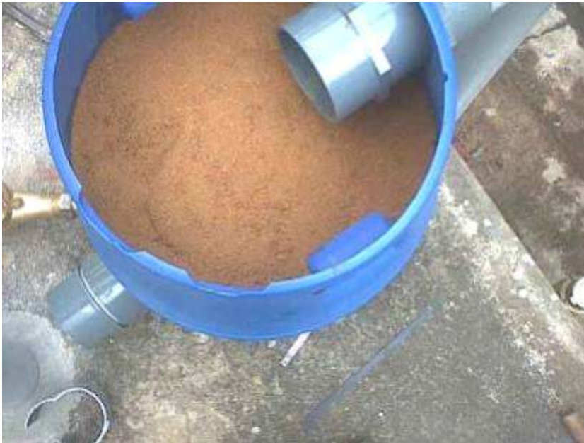
Drum filter filled with sand
