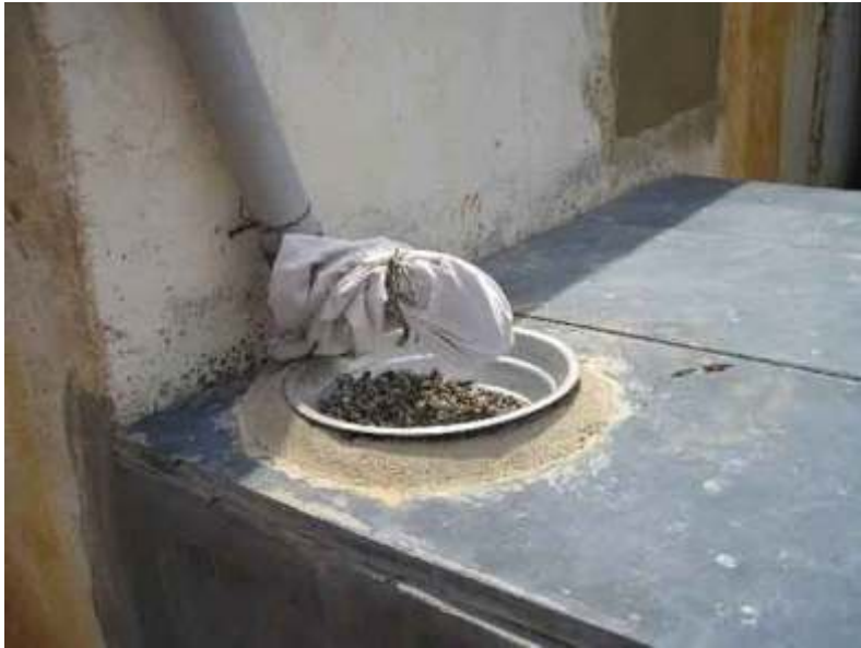
Filter with cloth tied to pipe and gravel in a perforated aluminum vessel
