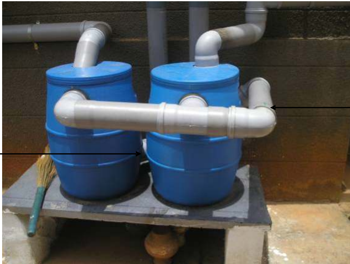
Drum filter for the roof top harvesting system of an apartment
