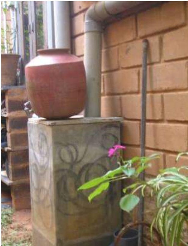
Ferro cement filter
