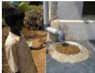
Integrated sand filters
