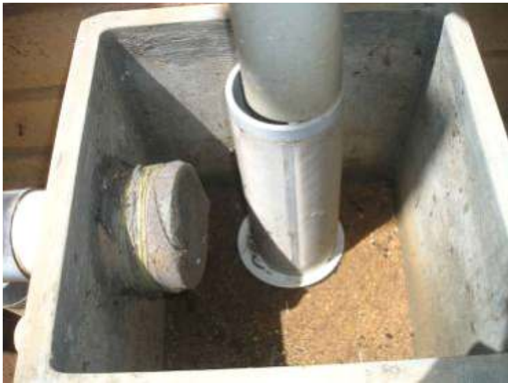
Ferro cement filter with sand
