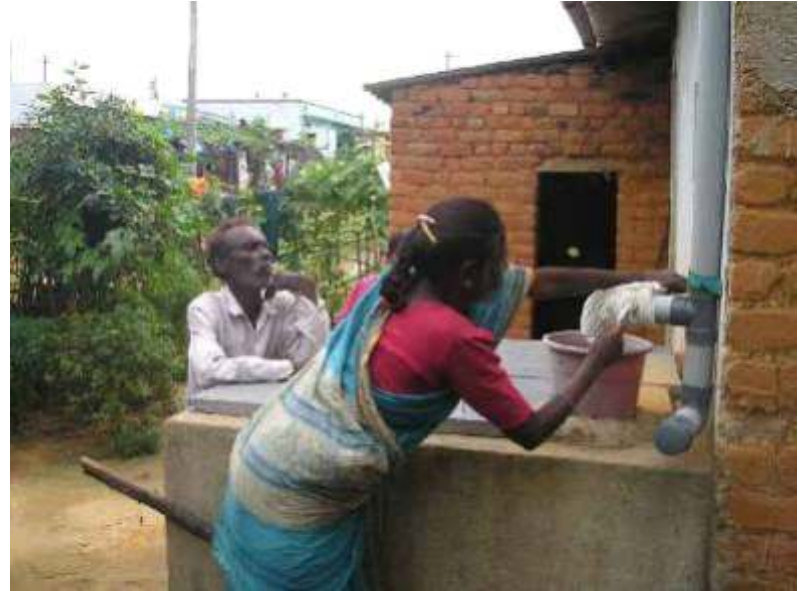
Woman placing a clean cloth filter on the pipe
