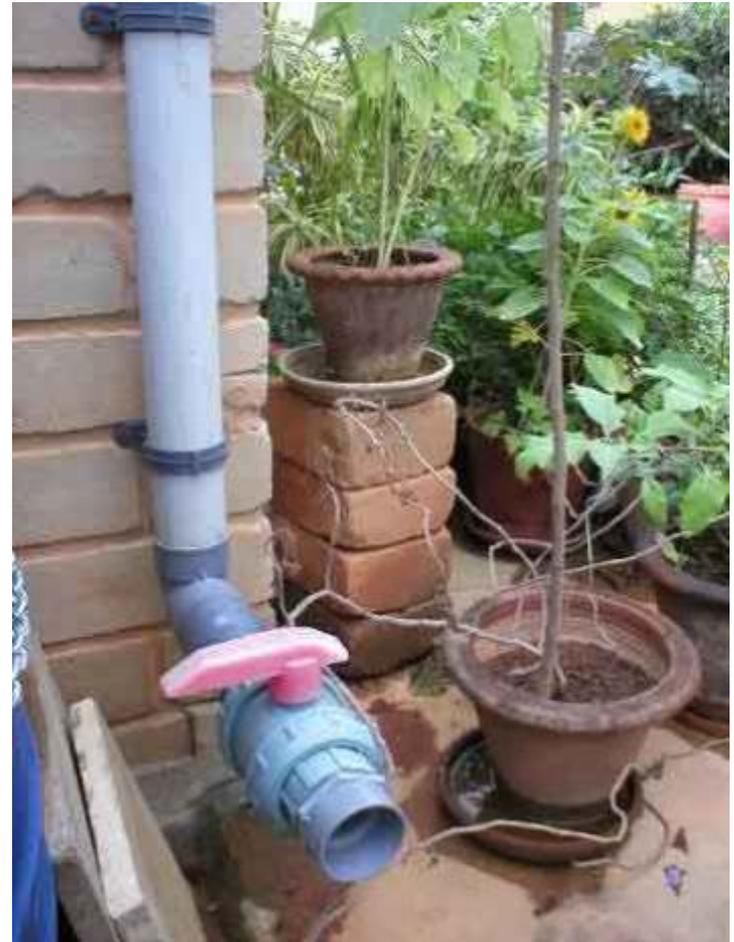
First rain separator with gate valve
