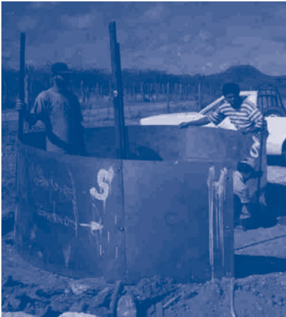
Screwing together the steel sheet form
