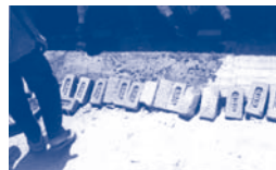
Laying mortar on mesh
