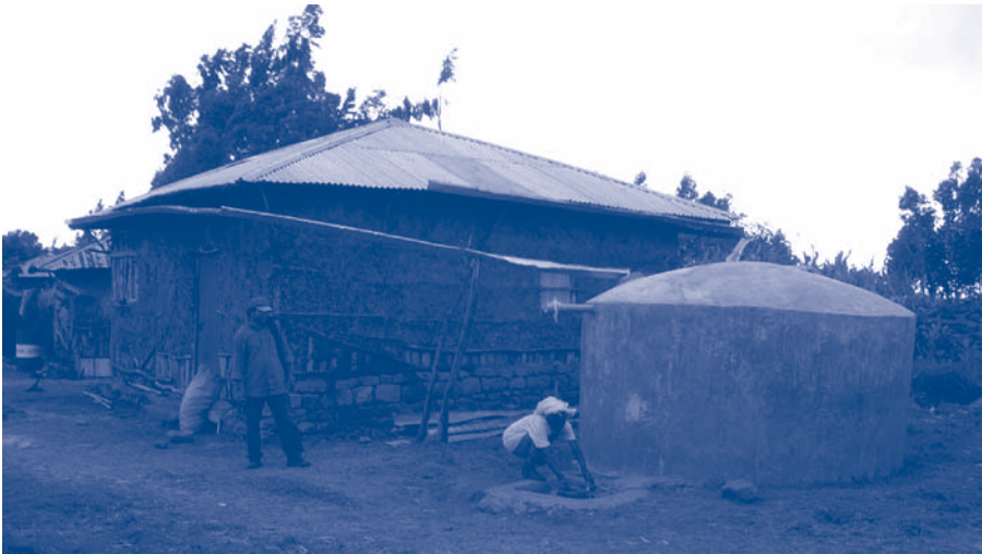
Figure 7.3. Typical rural building in Ethiopia with an unsustainably costly ferrocement tank (Picture: B. Woldemariam)
