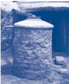
Burned brick tank in rural Uganda (Picture: V. Whitehead)
