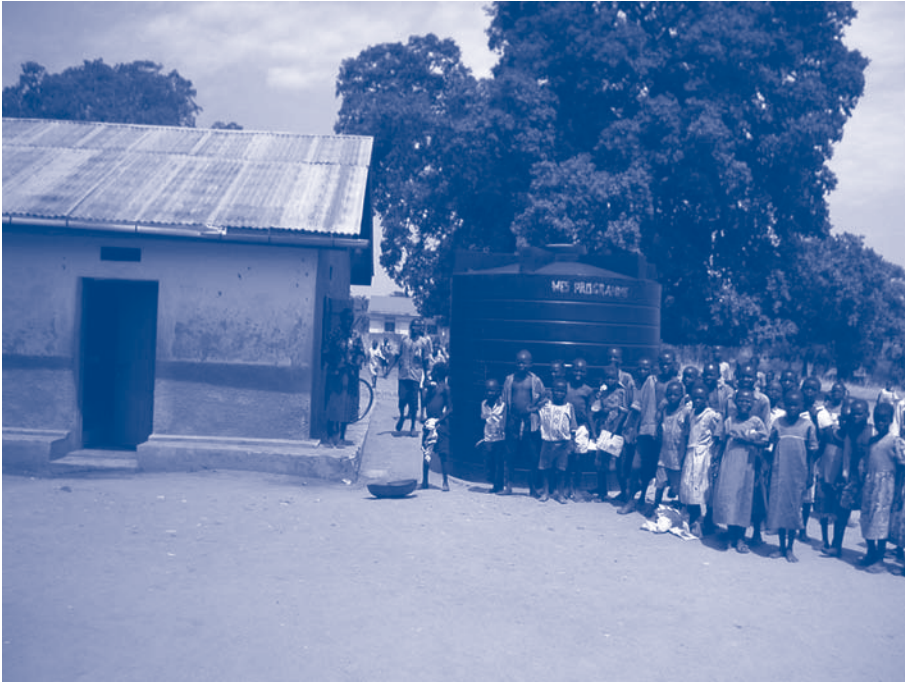
Figure 10.1. Unworkable school system in NW Uganda (Note entrance to the plastic tank is above gutter level)
