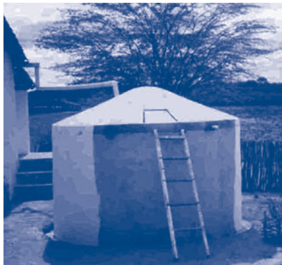
Finished tank being painted
