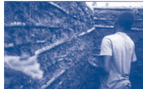
Daubing the walls
