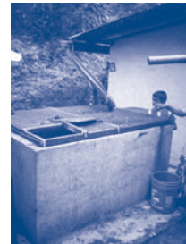
A plastered rectangular brick tank in rural Sri Lanka (Picture: D. Rees)
