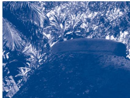
Detail of access to tank
