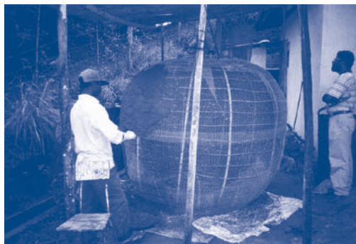
Partially rendered tank
