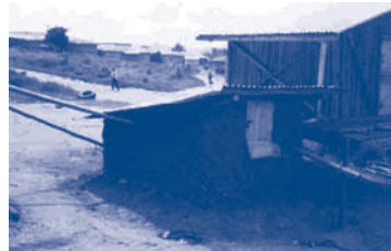
Completed tank (Pictures: D. Rees)
