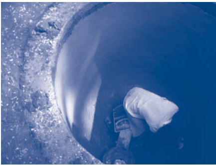
Lining the pit
