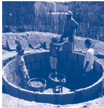
Fixing the plates
