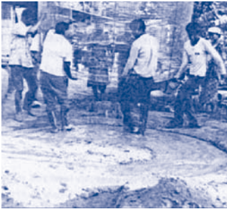
Moving the mould into place
