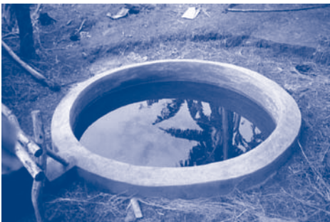
Underground tank with sloped ring beam
