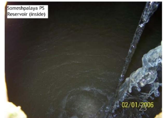
Figure 9: Water being pumped to Someshwarahpalya reservoir
