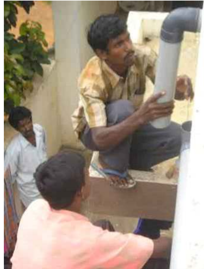
Connecting vertical pipes
