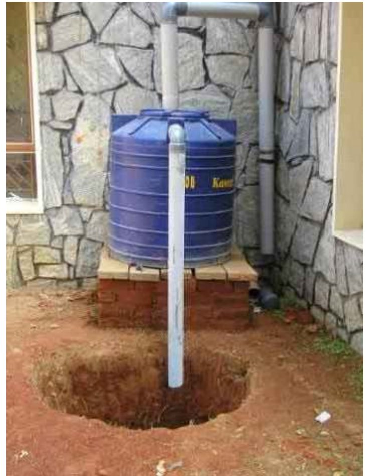
Overflows from rain barrels can also be used for recharging the groundwater
