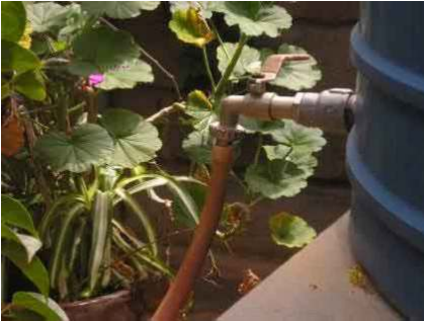
Using a hosepipe, the tap can be connected to the borewell or sump tank.
