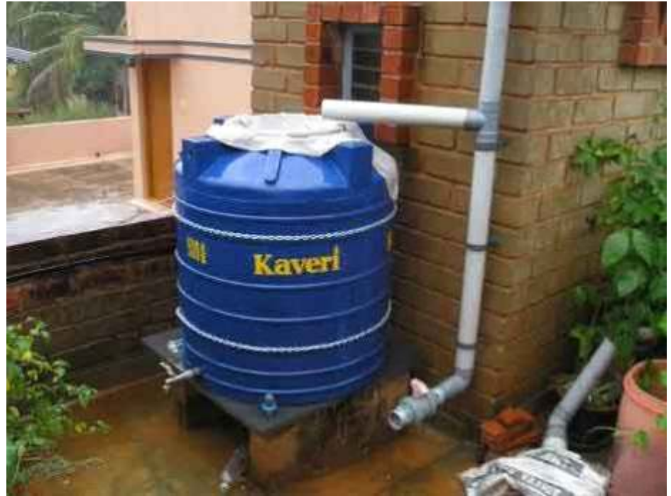
A 500 liters rainbarrel at work on a roof
