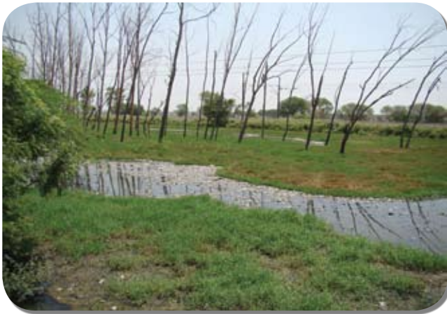
Pic 9: Waste water from Gannaur town (Sonapat) accumulated along the railway track. Trees have dried as a result. 17.6.10
