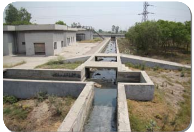
Pic 14: Idle 35 MLD STP at Panipat. 29.4.10
