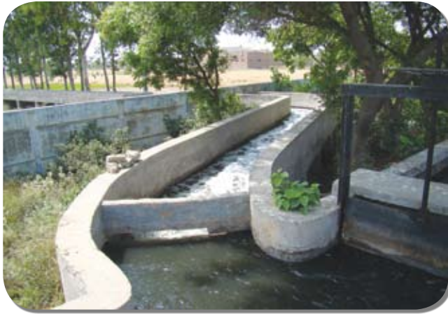
Pic 11: Poor quality Effluent from 10 MLD STP at Panipat. 12.4.10
