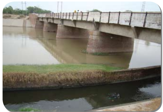
Pic 20: Drain no 6 (foreground) carries waste water to the river alongside Drain no 8 that supplies drinking water from WYC to the WTP at Wazirabad (Delhi). 16.6.10
