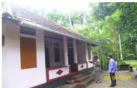
Water falling on the roof is collected through a PVC gutter and diverted through a pipe to the domestic open
