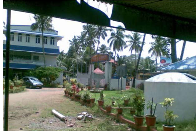
Rainwater falling on the multi-storied building at KIDS campus is collected and diverted to the well, which is given a tank like coverage structure above ground. The quality of water in this well and surrounding areas drastically improved as a result of this measure. KIDS attempted injection of rain water from a 600 square feet auditorium in to a large contaminated well in their own campus in 2005, taking advice from Mr. Terry Thomas of PLANET Kerala. This turned out as remarkable success. Water quality of this contaminated well and other wells in its vicinity improved. This is a clear example of how injecting rainwater in to one large well could influence the near by areas. The process of quality improvement of water is more effective if the soil is mostly sandy in nature. Back washing is most effective, in the sandy soil as the water could move through the interstitial space of the sandy soil, flushing out the excess nutrients and contaminants found in its midst.
