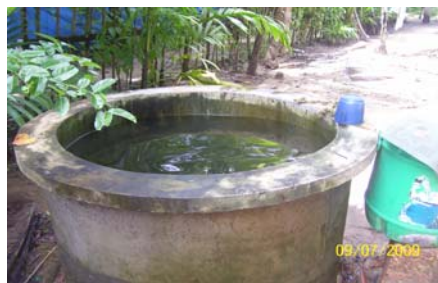
Water falling on the roof is collected through a PVC gutter and diverted through a pipe to the domestic open
