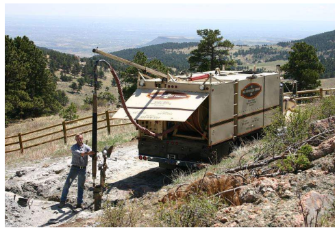
Fig- 5, Packer Installation.
